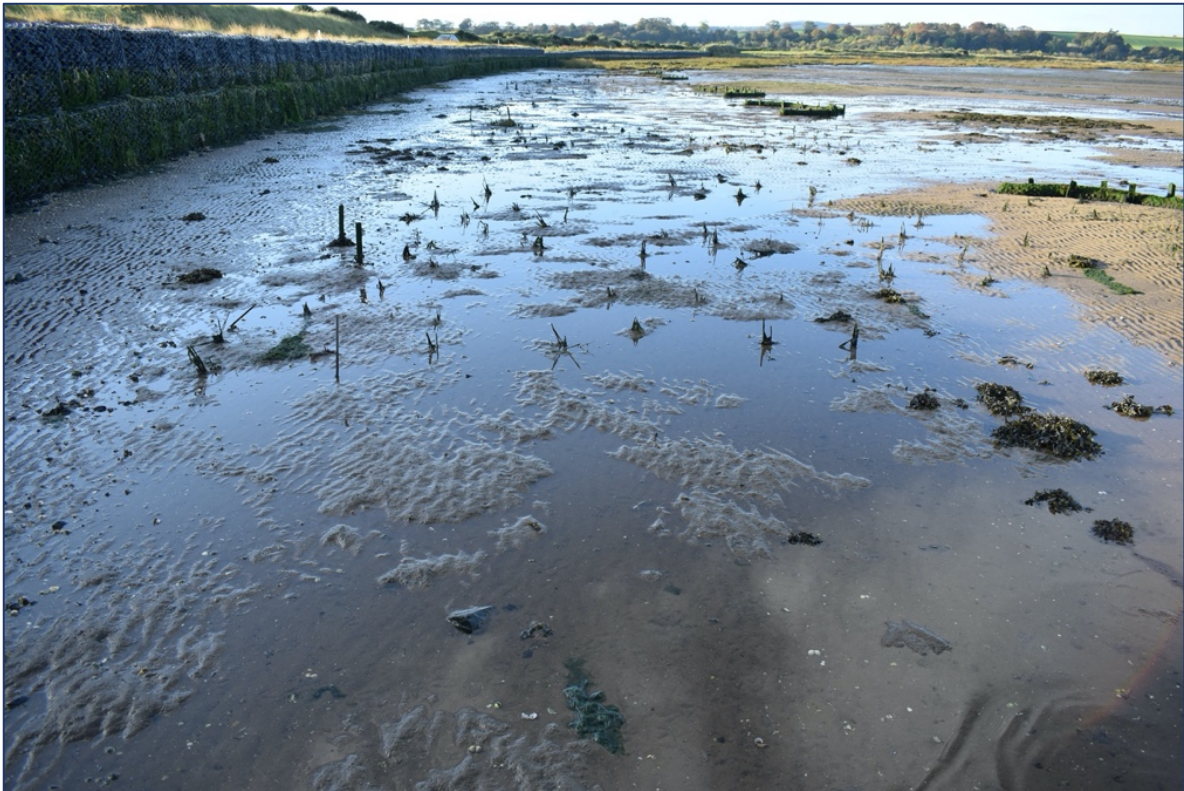
Figure 15. Bio-rolls have assisted the process of sedimentation on the mudflats, Eden Course, 2018.
