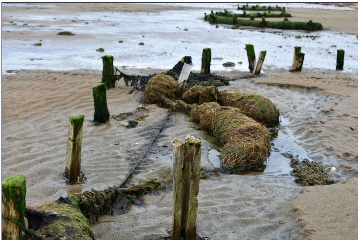
Figure 18. Irreparable storm damage to bio-rolls at Dornoch Sands, 2018.
